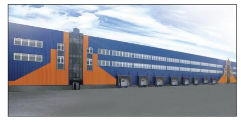
The building is divided into six independent sections (each at least 6,400 sq m), with internal clear ceiling of 12m height and industrial flooring constructed with anti – dust overlay quartz finish. The terminal accommodates 90 parking spaces for cars and trucks, as well as 24 hour security and municipal provided sewage, water and garbage collection.
