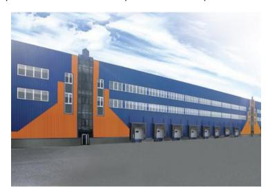
The building is divided into six independent sections (each at least 6,400 sq.m.), with internal clear ceiling of 12m height and industrial flooring constructed with an anti – dust overlay quartz finish. The terminal accommodates 90 parking spaces for cars and trucks, as well as 24 hour security and municipal provided sewage, water and garbage collection.
